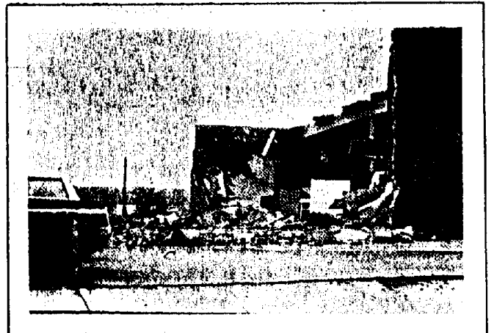
Even reinforced masonry failed similarly to tilt-up walls in the 1971 San Fernando earthquake in the industrial buildings.
