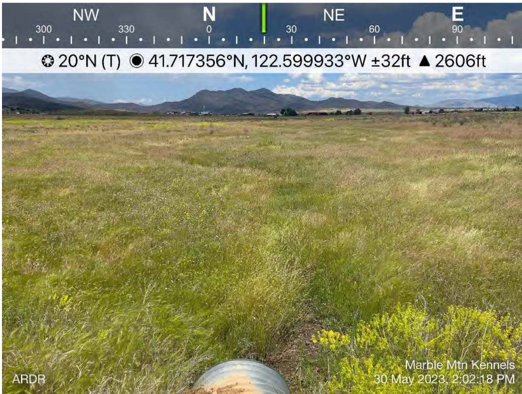
Photo 2. MM Kennels NW Parcel seasonal drainage exiting culvert at access road
